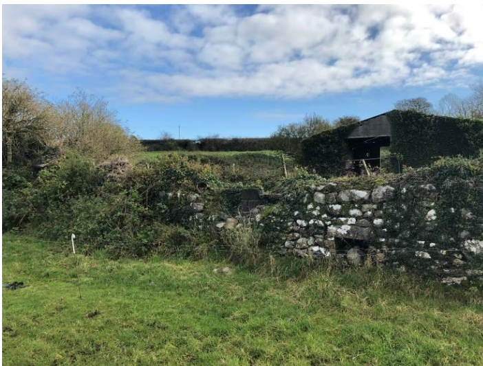
Plate 11.7: Remains of vernacular farmstead (CH 1), facing east-northeast
