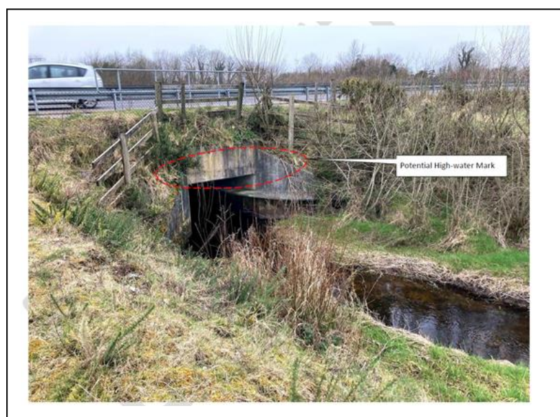
Insert 6.2 Culvert under M81 motorway.
