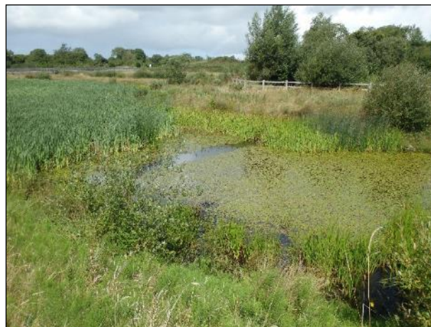
Plate 2 Existing attenuation pond of the M18 Motorway dominated by various macrophytes species
